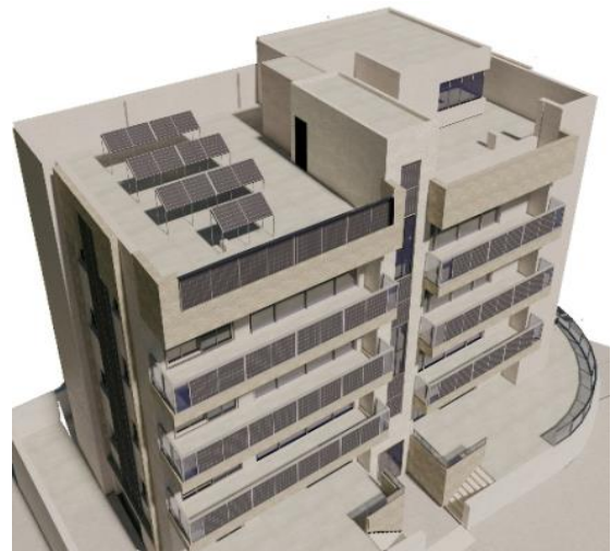
Figure 14. Roof PV panels distribution
