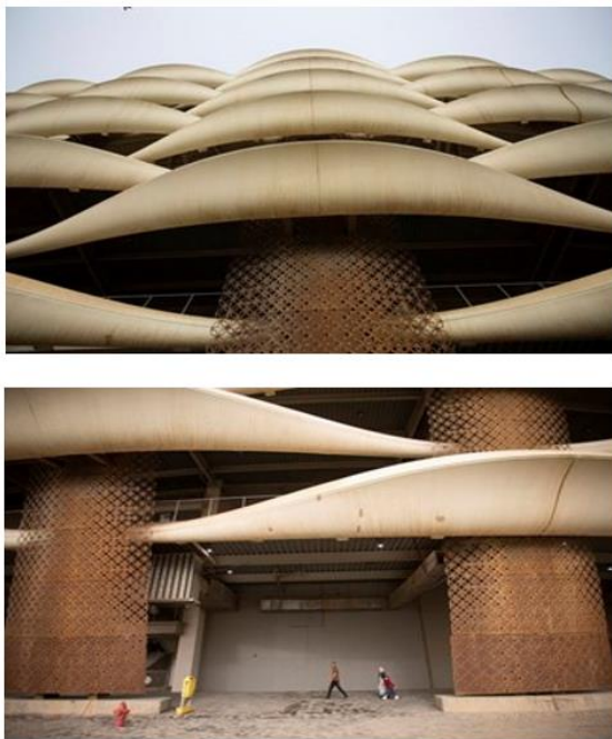
Figure 1. Sports City project in Basra
