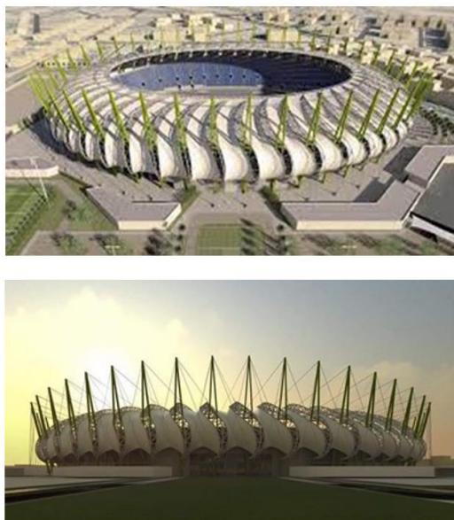
Figure 2. Mina Stadium project in Basra
