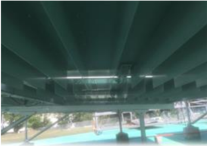
Figure 1. The backside of the experimental PV setup
