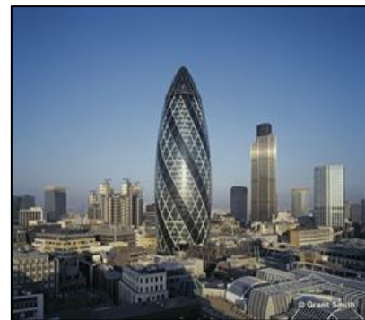
Figure 3. An office tower of 30 St Mary Ax in London
