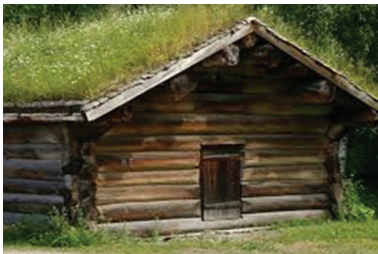
Figure 4: Old cogged house.
