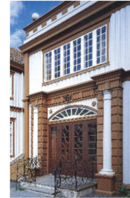
Figure 22: Leangen Imitated hewn stone.
