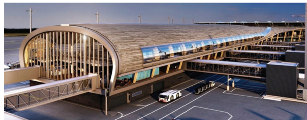
Figure 28: Oslo Airport, new pier.
