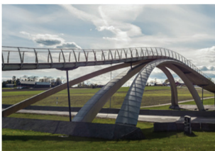
Figure 29: The da Vinci bridge, Ås, (2001).
