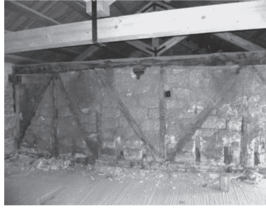
Figure 7: Wooden partition wall where spaces are filled with reed.
