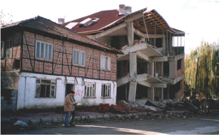
Figure 14: A humuş standing next to a destroyed contemporary reinforced concrete construction after the Düzce earthquake in 1999 (yoremizden.com).
