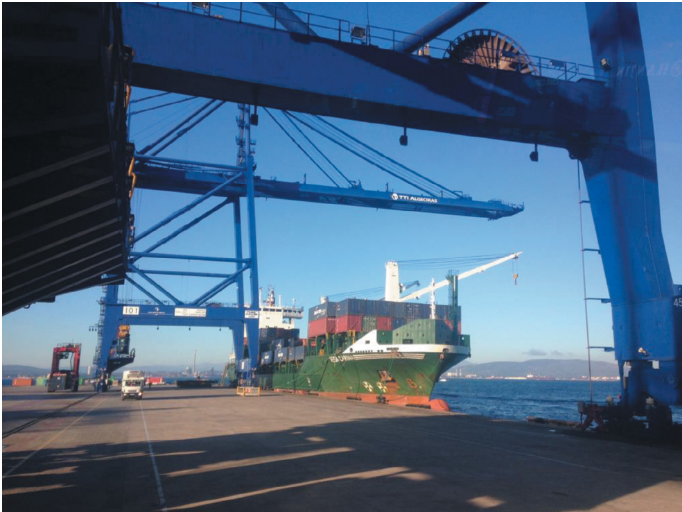
Figure 1: Container terminal in Algeciras port.
