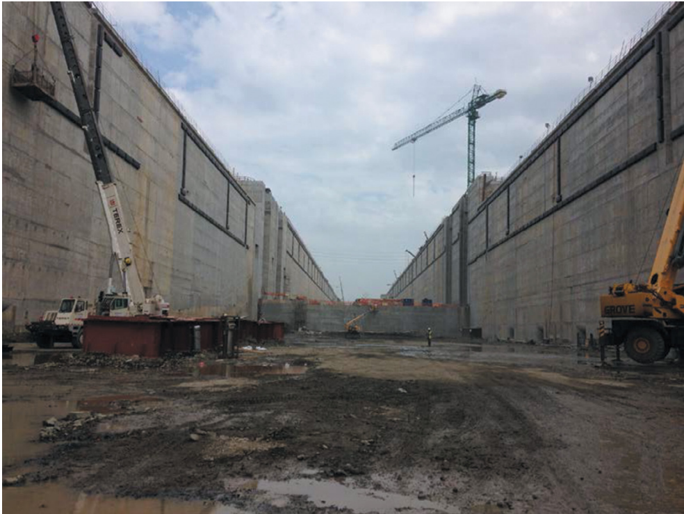
Figure 3: Third set of locks in Panama Canal expansion project under construction.
