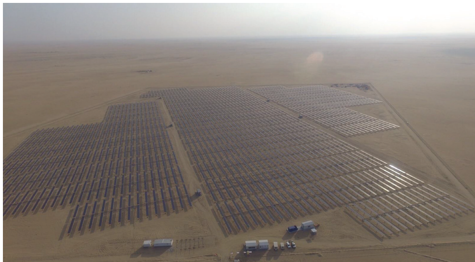
Figure 7: Aerial view of Sedra project. Mina Al Ahmadi
