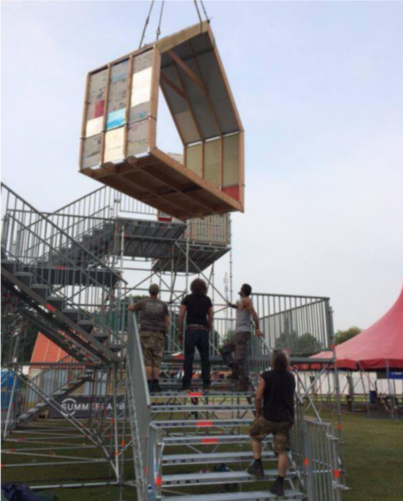
Figure 4: Placing a structure on the tower of scaffolding.
