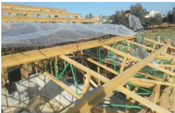
Figure 16: Installing roof insulation.
