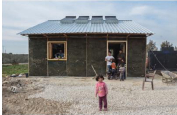
Figure 20: Completed school unit.
