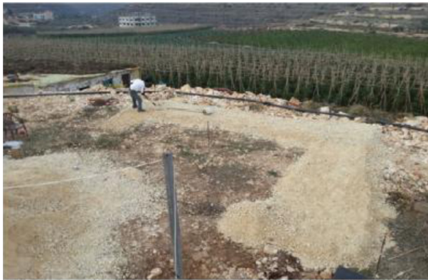
Figure 3: Site preparation & leveling.
