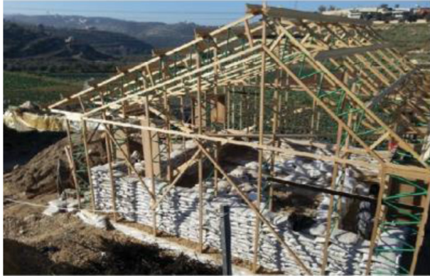
Figure 14: Assembling roof structure.
