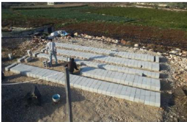
Figure 4: Assembling earth ducts.
