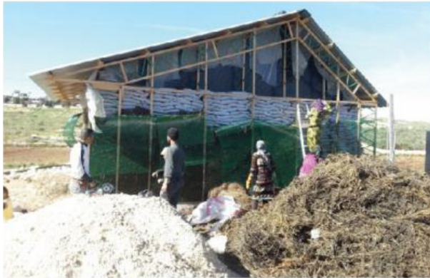
Figure 18: Filling with insulation.
