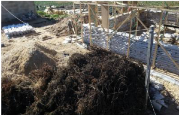
Figure 15: Collecting insulation material.
