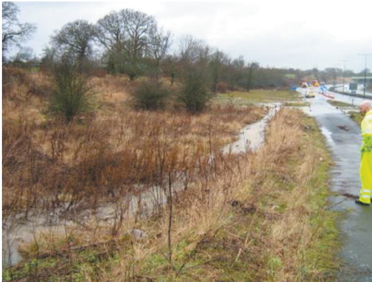
Figure 2: Photo of flood water running down from the Bushey Heath urban catchment onto the carriageway on 11–15th January 2008, facing north.
