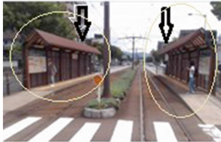
Figure 3: Sidewall of train stop.
