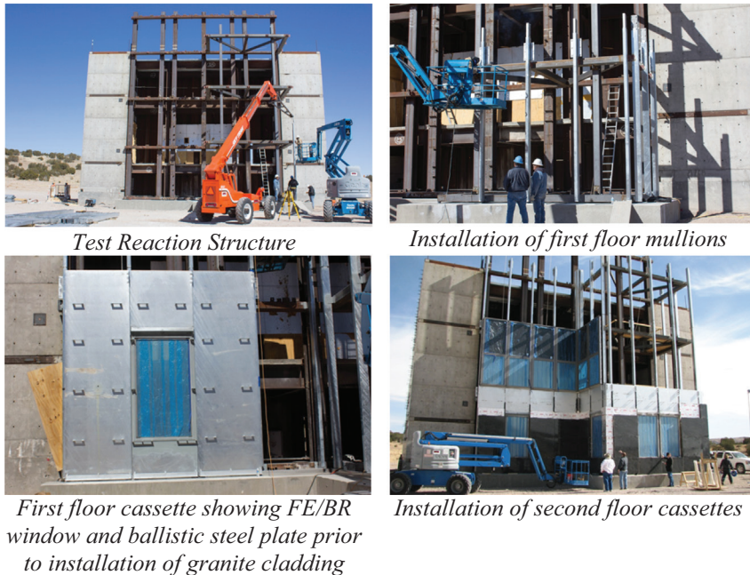
Figure 3: Installation of SSCW test structure.
