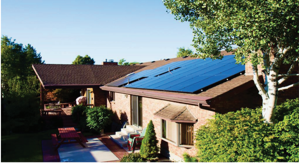
Figure 2: View of entire solar panel on the roof of a Boise, Idaho, area home. Photo courtesy of Blue Raven Solar Systems, Salt Lake City, Utah.
