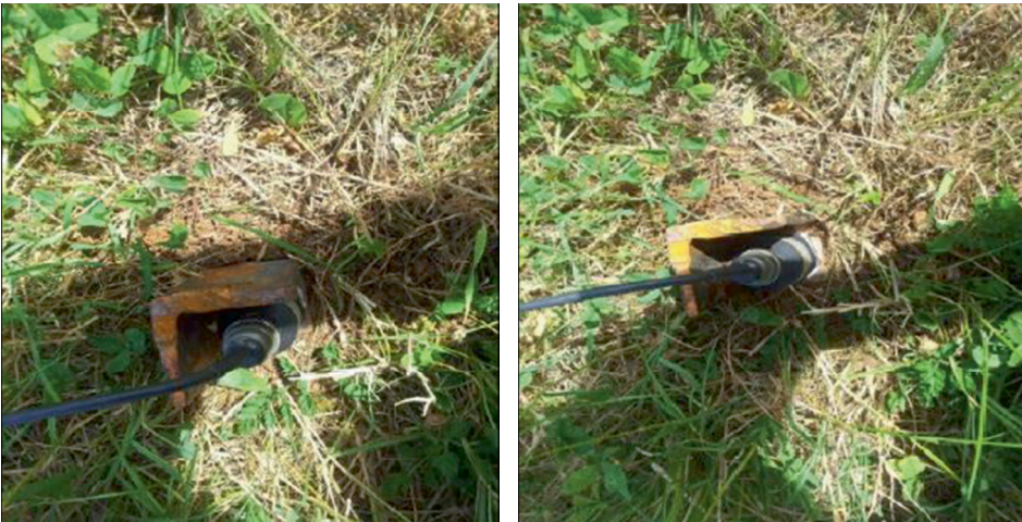
Figure 4: Accelerometer fixed on steel spikes.
