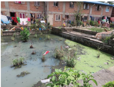
Figure 5: Kirtipur upper constructed wetland in the September 2018.
