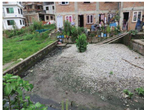
Figure 6: Kirtipur upper constructed wetland in the September 2019.
