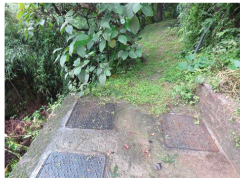
Figure 10: Place of the not well-functioning constructed wetland at Chandra Ban Eco Resort, September 2019.
