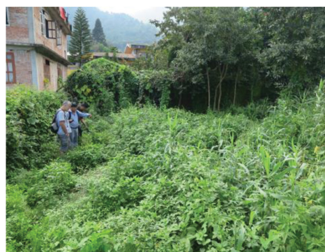
Figure 8: Shuvatara school semi-functioning constructed wetland, September 2018.
