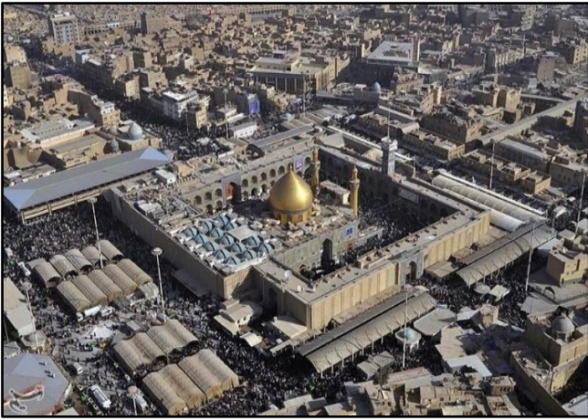
Figure 9. Building design cars in An-Najaf traditional city
