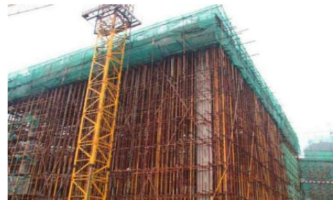
Figure 8. Modern formwork systems use formwork made of iron
