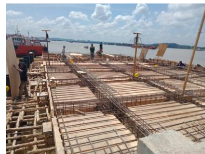
Figure 3. Formwork installation process
