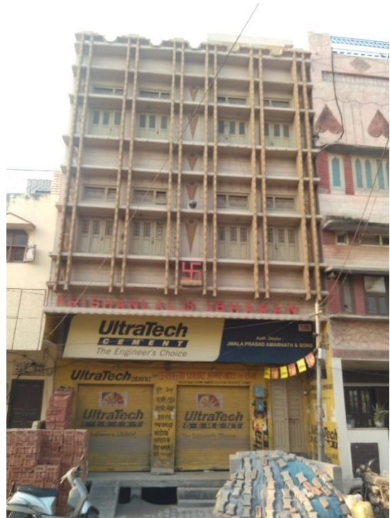
Figure 11. Shading devices seen on the front facade of a shop-cum-houses
