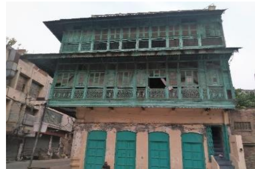
Figure 1. A typical three-storey high shop-cum-house in Ambala
