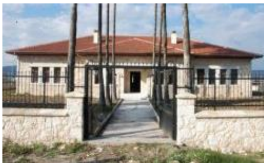
Figure 23. Current State of Silifke Tekir Farm [21]
