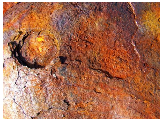
Figure 1. Effect of atmospheric corrosion on metallic surfaces
