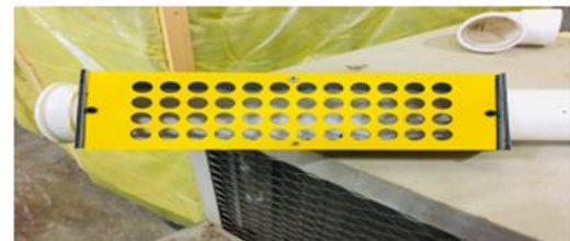
Figure 6. Air outlet supplying for ventilation (PV) diffuser
