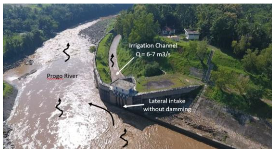
Figure 4. Lateral intake without damming (Aerial photo of DJI Phantom 4 UAV)
