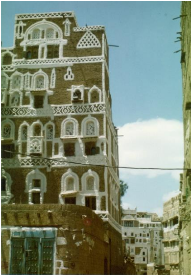
Figure 13. The Traditional House (Tower House) in Sana'a City
