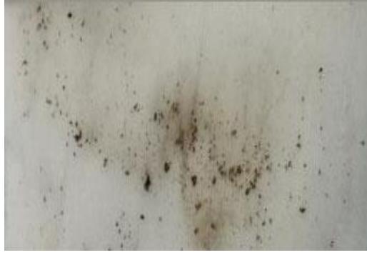
(b) Rock particles fell off after freeze-thaw cycles
