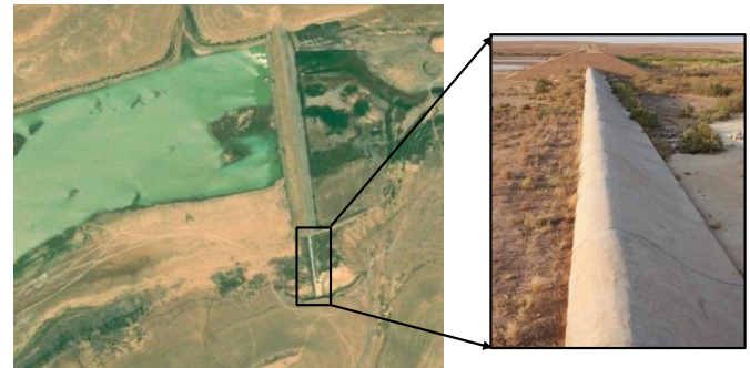
Figure 1. An aerial image of H2 Dam with a photograph of the spillway
