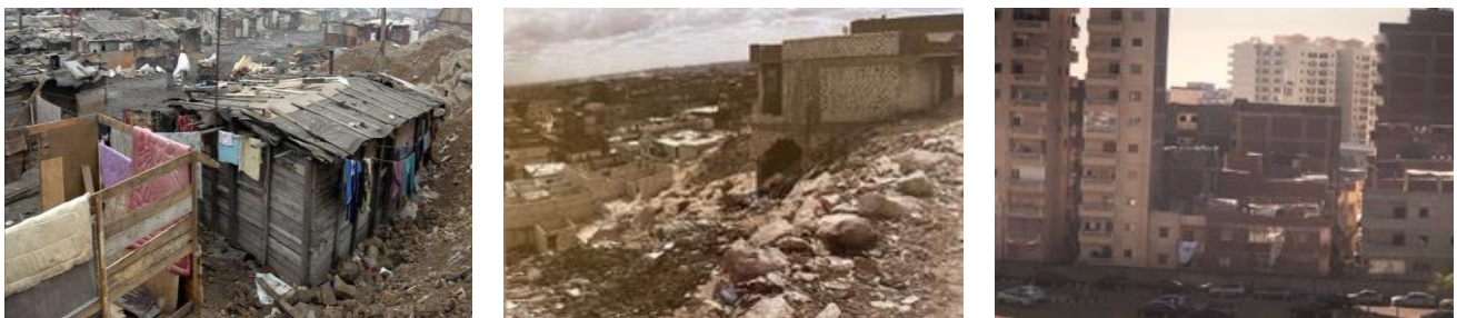
Figure 2. Slums as unsafe overcrowded houses
