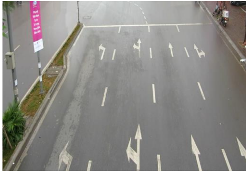
Figure 4. Stop lines on the road
