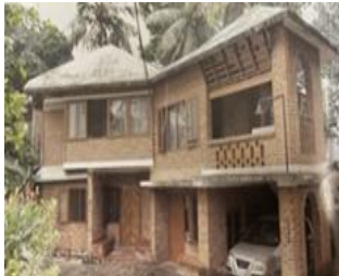
Figure 11. Subrahmaniam House Source: Untold stories, Laurie Baker Centre
