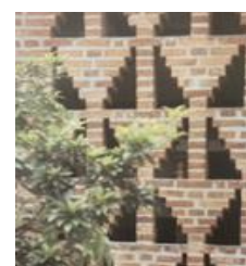
Figure 9. Jalli work pattern in George house Source: Untold stories, Laurie Baker Centre
