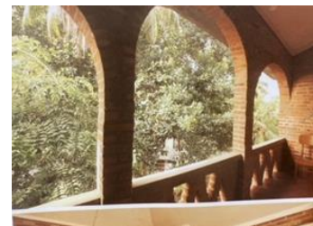
Figure 16. Verandah overlooking lake in George house. source: Untold stories, Laurie Baker Centre
