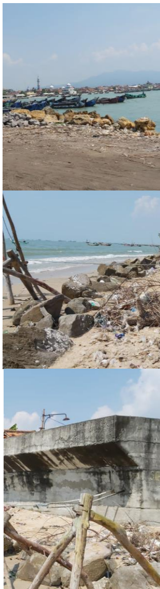
Figure 12. Structural mitigation performed by the community
