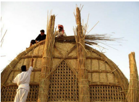
Figure 3. Teamwork houses construction [13]
