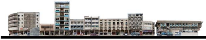
Figure 3. The current state of the façade of the Rasheed Street wall overlooking the south in Bab Al-Sharqi [1]
