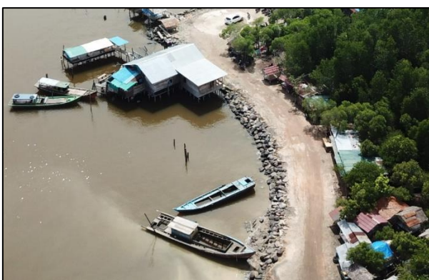
Figure 3. The revetment building with a dump stones system in Bandar Bakau Dumai (Source: Aras Mulyadi Personal Documentation Year 2020)
