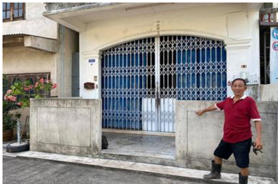
Figure 4. Flood barriers were constructed to prevent the water flow in PTSM
