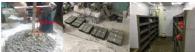
Figure 2. Preparation of concrete test pieces
