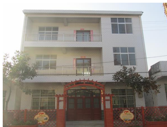
Figure 2. A typical brick-concrete building in the study area
