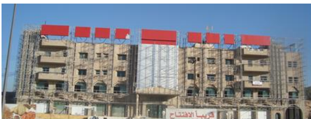
Figure 3. The use of Alucobond cladding instead of limestone. Source (researcher)
