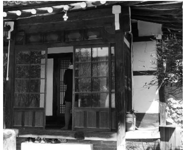
Figures 6. Screen walls and panels at a guesthouse currently in use in Hwangnamdong, Gyeongju, South Korea
