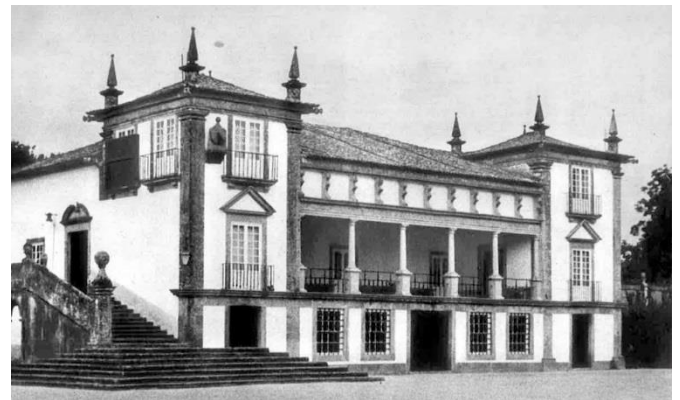
Figure 1. Solar de Bertandos (Ponte de Lima), one of the baroque manor houses documented in the Inquérito
