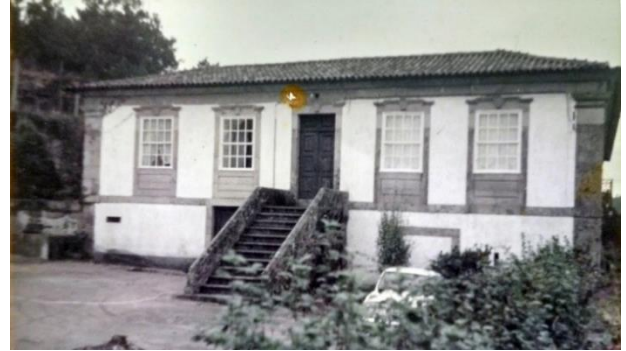
(a) State prior to intervention
