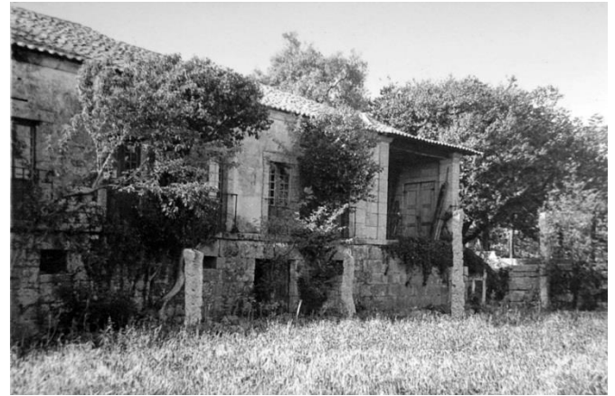
(a) State prior to intervention (Courtesy of J.B. Távora)
