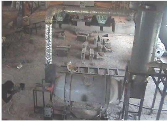
Plate 9: Furnace being test run with recuperator (Temperature being measured with optical pyrometer)
