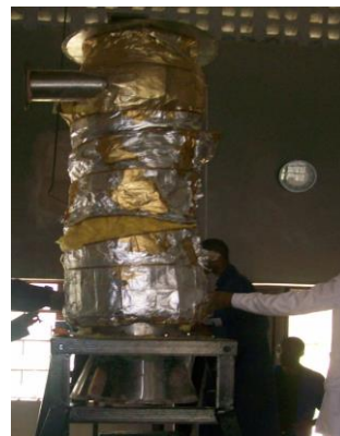
Plate 7: Recuperator assembly installation in Progress - 1
