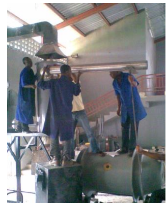
Plate 8: Recuperator assembly installation in Progress - 2
