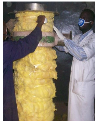
Plate 5: Recuperator assembly being lagged
