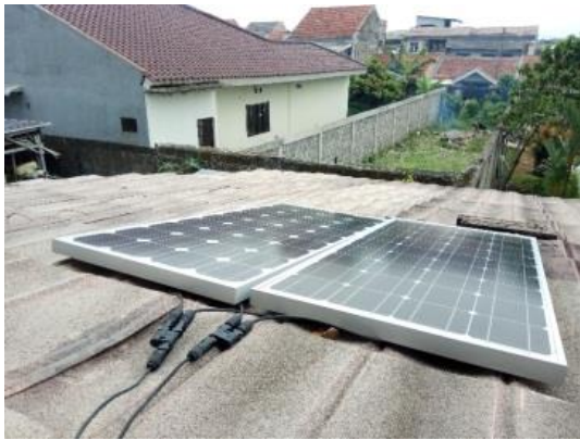
Figure 9. Installation of Photovoltaic.
