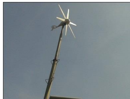
Figure 8. The Mini power plant with windmill installed
