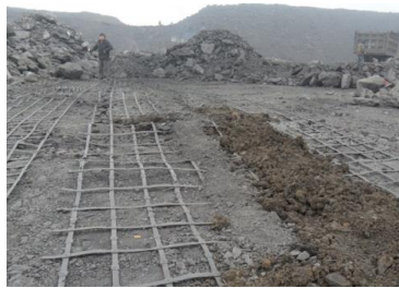
Figure 3. Geogrid arrangement
