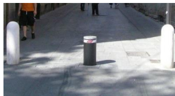
Figure 10. Retractable mobile barriers
