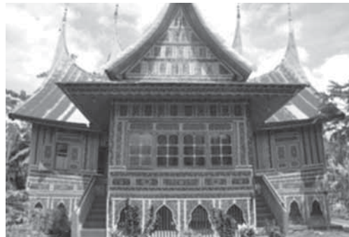
Figure 2: Datuk Paduko Alam house Nan In Lintau Buo, Tanah Datar.
