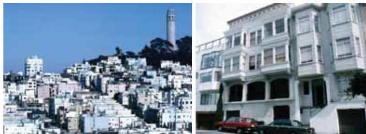
Figure 13: Vernacular town housing in San Francisco, USA.
