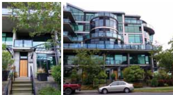
Figure 15: Contemporary town housing built at street level for effective surveillance with apartments above, Victoria, Canada.
