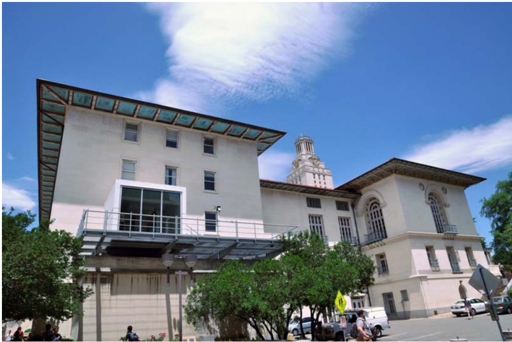
Figure 1: View of Facade Laboratory on platform.
