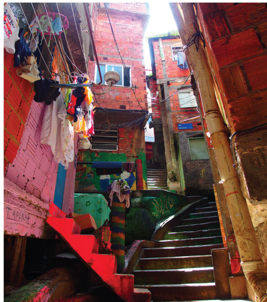
Figure 2: Informal “street” of Santa Marta favela in Rio de Janeiro, photo: RB.
