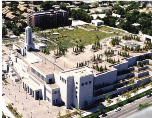
Figure 2: LDS Conference Center in downtown Salt Lake City is host to a Hydrotech intensive green roof system.
