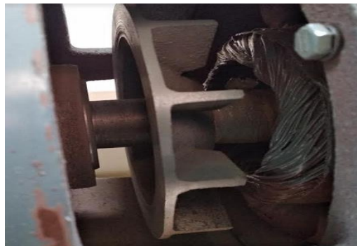
Figure 5. Shaft connected to generator with bearings
