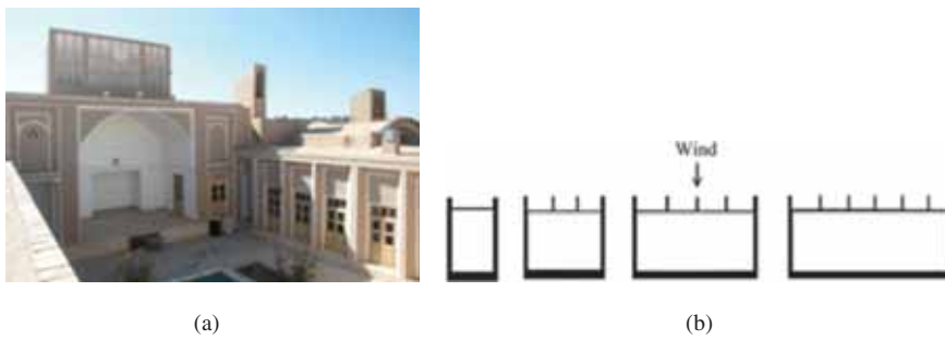
Figure 3: One-sided (Ardakani) badgir : (a) a house in Ardakan and (b) typical plans.
